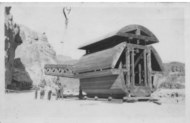
Above: This "animal" postcard depicts a construction machine designed and built to fill 18 feet diameter tunnels with concrete. Unknown date and location, but this RPPC is valued at $34.
