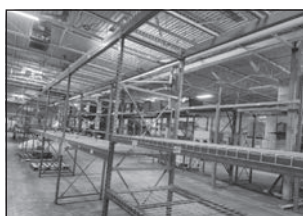
Lots of Pallet Racking
